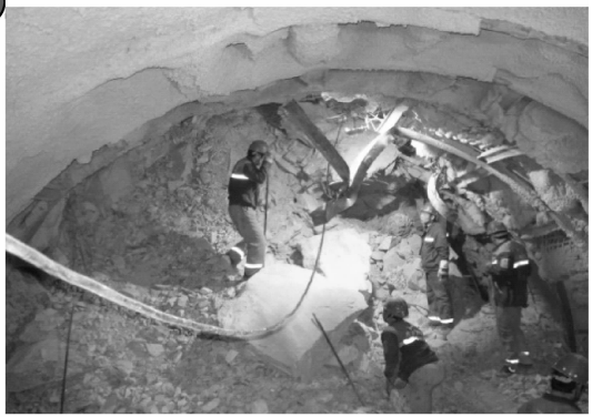
(b) Rock burst causing the falling off of bolts
